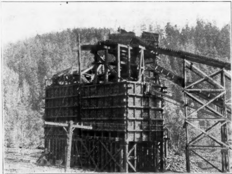
The Plant of the Western Sand and Gravel Company
